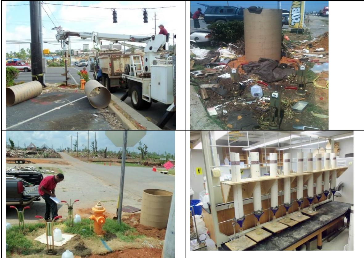
Figure 4. Photographs showing borehole drilling, Sonotube infiltration tube installation, double-ring infiltration measurements, and laboratory column tests.
